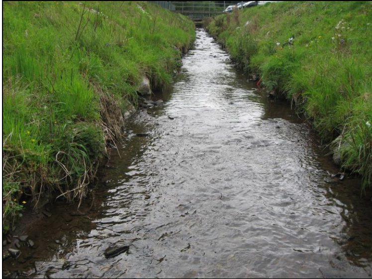
Plate 1: Grange Stream western open section in Donnybrook Commercial Park, looking west
