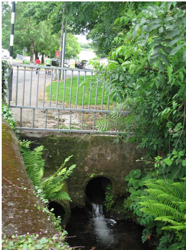
Plate 15: Tramore River emerging from culvert under Brook Avenue, looking south
