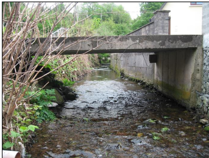
Plate 9: Middle Ravensdale Bridge on Ballybrack Stream, southern elevation
