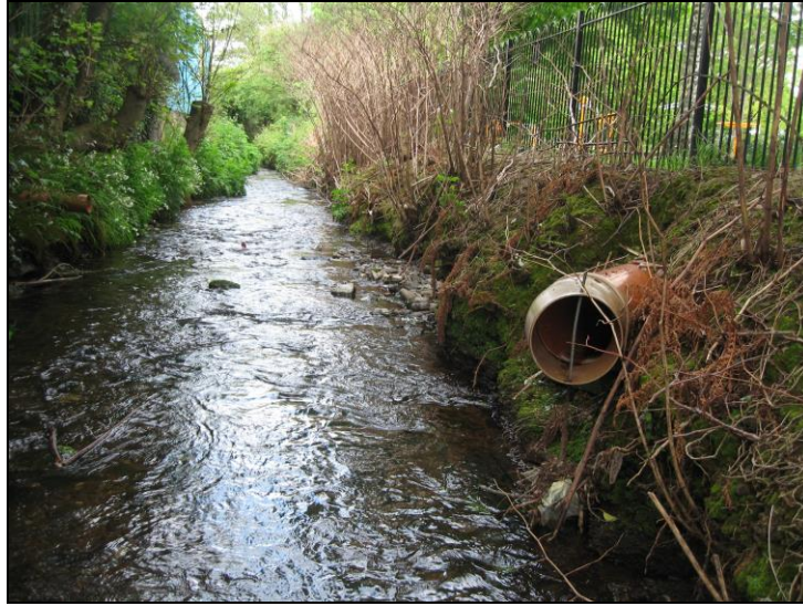
Plate 4: Ballybrack Stream, Douglas Community Park, looking north
