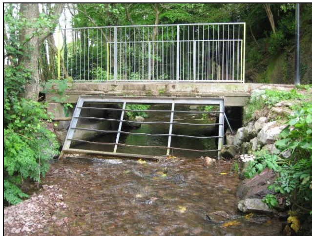
Plate 12: Ballybrack Stream showing bridge and trash screen in Ballybrack Woods, looking south
