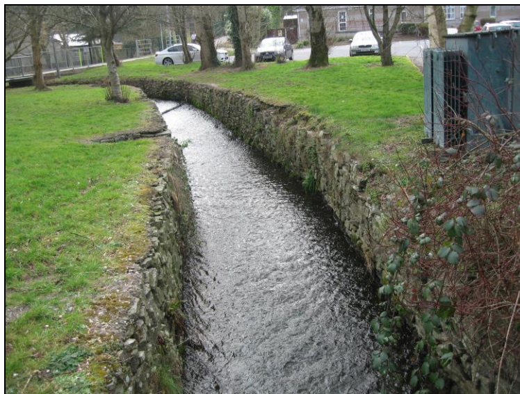
Plate 6: Ballybrack Stream, looking southeast with bridge to Ballybrack Woods in background
