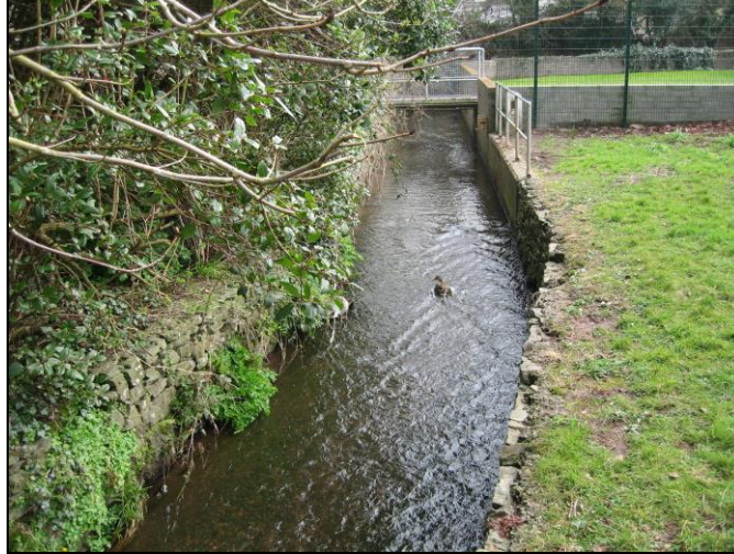
Plate 7: ICA Bridge on Ballybrack Stream eastern elevation
