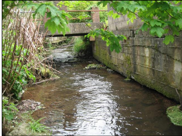
Plate 10: Upper Ravensdale Bridge on Ballybrack Stream, northern elevation
